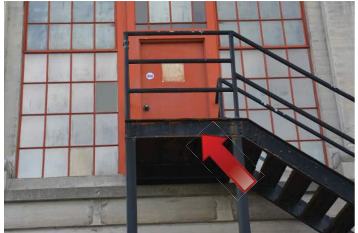
Door and stairwell on the second floor of the east elevation. Image by Otak. 200224 CoT CAS EL-E DSC_1039.JPG
