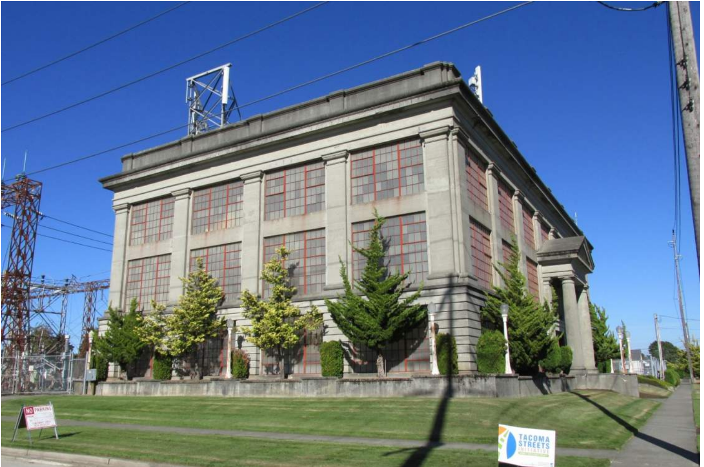
Figure 18 Cushman Substation, view northeast
