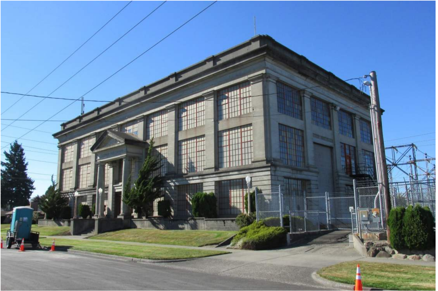
Figure 17 Cushman Substation, view northwest.
