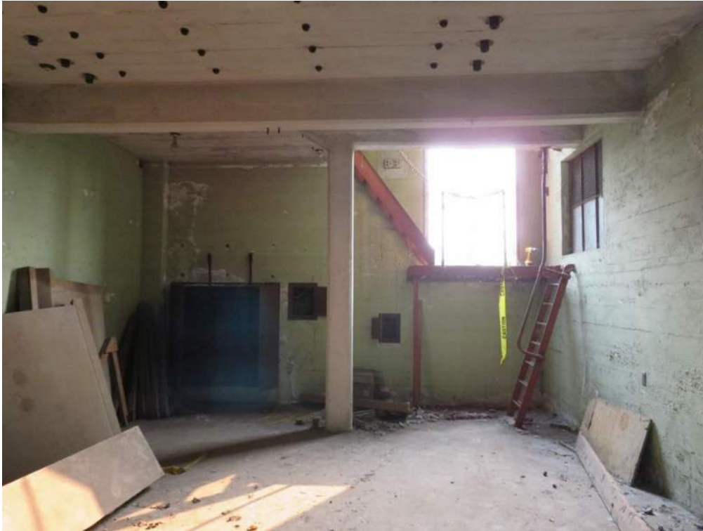
Photo 8 of 13. WA_PierceCounty_AdamsSt.Substation_0008. Adams St. Substation, interior, regulator room, lower level, view east.
