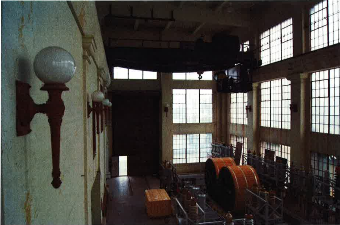
Photo 9 of 17. WA_PierceCounty_CushmanSubstation_0009. Interior of Cushman Substation, which is now used for storage. Note the decorative lighting, gantry crane (at ceiling), and voluminous interior space three stories high. Engaged pilasters are visible on both the south wall (pictured right) and interior wall (pictured left).
