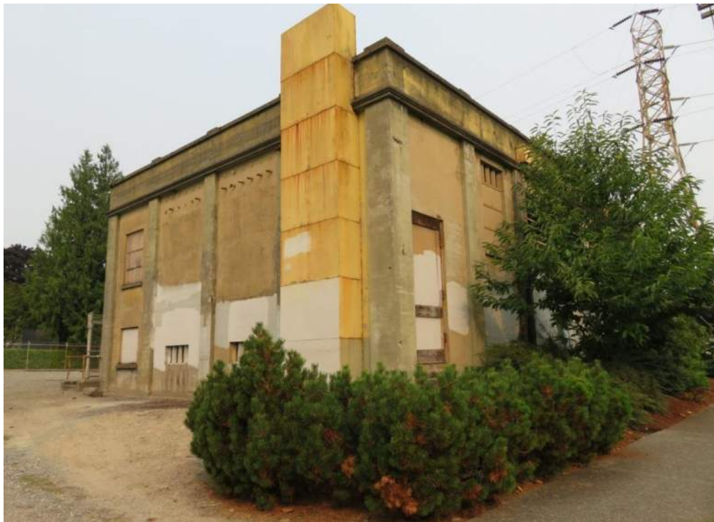
Photo 2 of 13. WA_PierceCounty_AdamsSt.Substation_0002. Adams St. Substation, oblique, view northwest.
