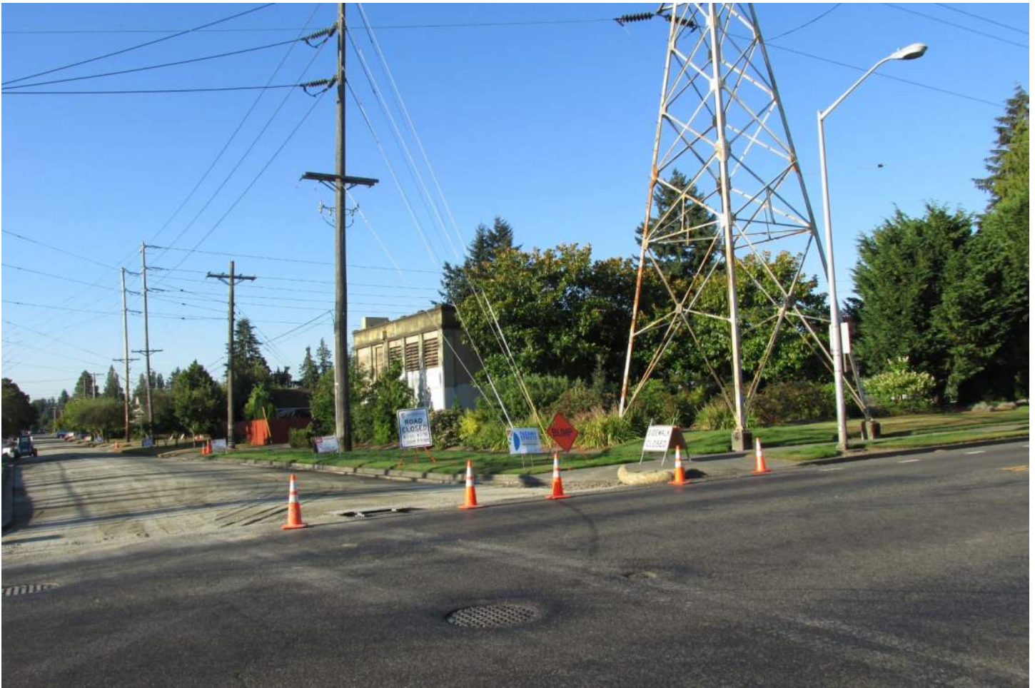
Figure 22 Adams Street Substation and Tower 1, view southwest
