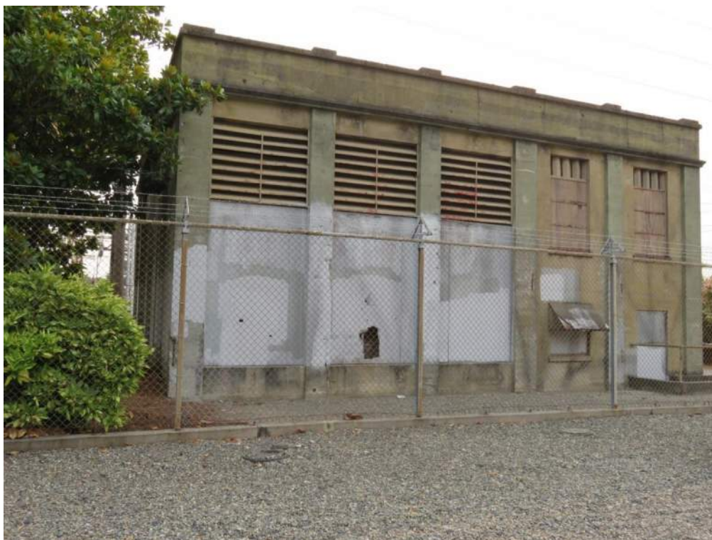
Photo 5 of 13. WA_PierceCounty_AdamsSt.Substation_0005. Adams St. Substation, west elevation, view southeast.
