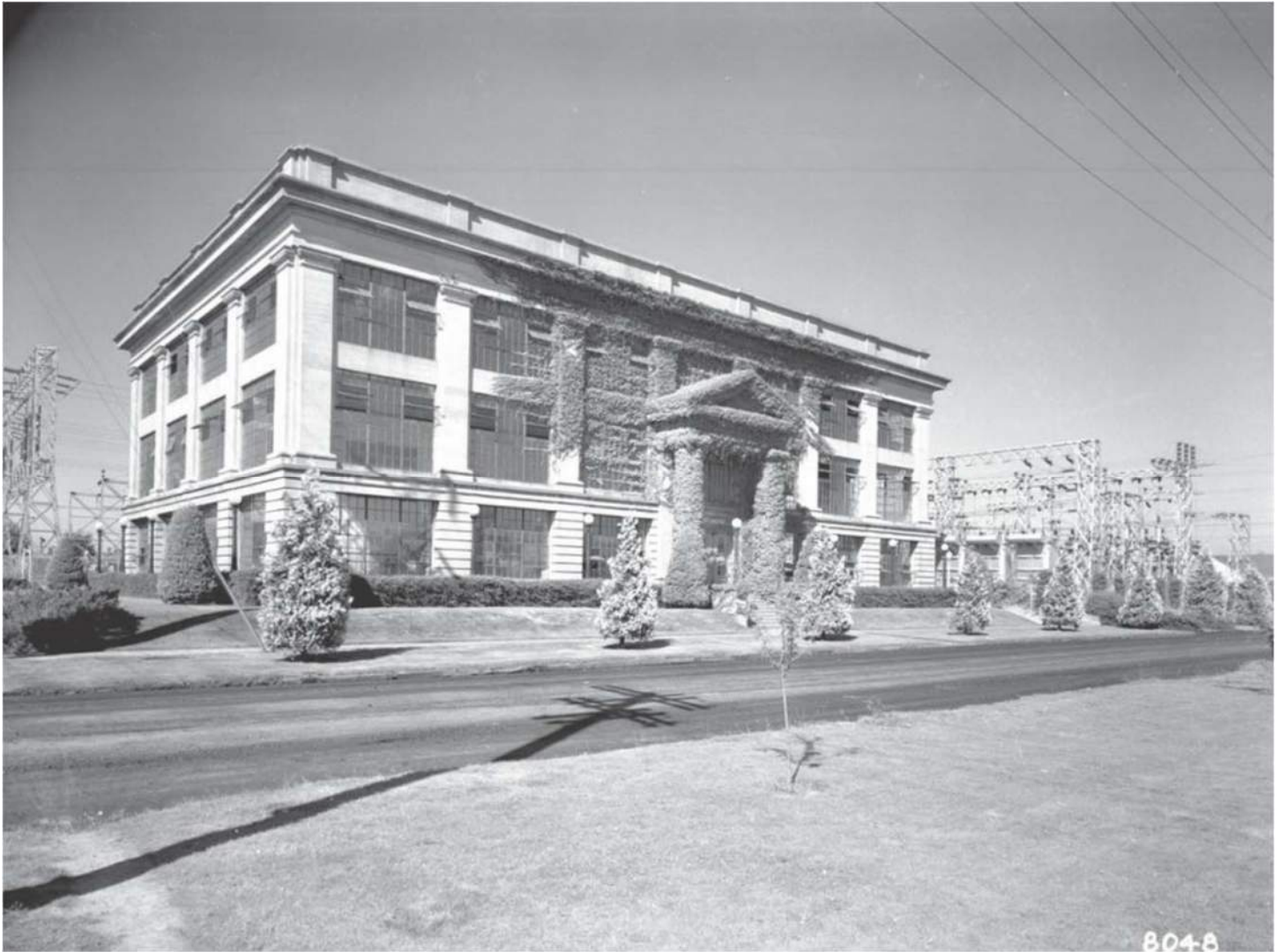
Figure 13 Cushman Substation, 19th Street facade, 1947, Image courtesy of Tacoma Power
