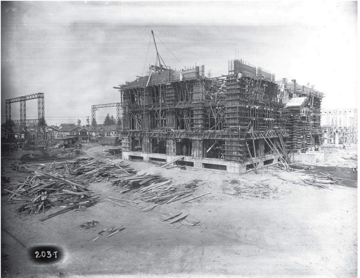
Figure 3 Cushman Substation under construction, board formed construction, August 3, 1925, Image courtesy of Tacoma Power
