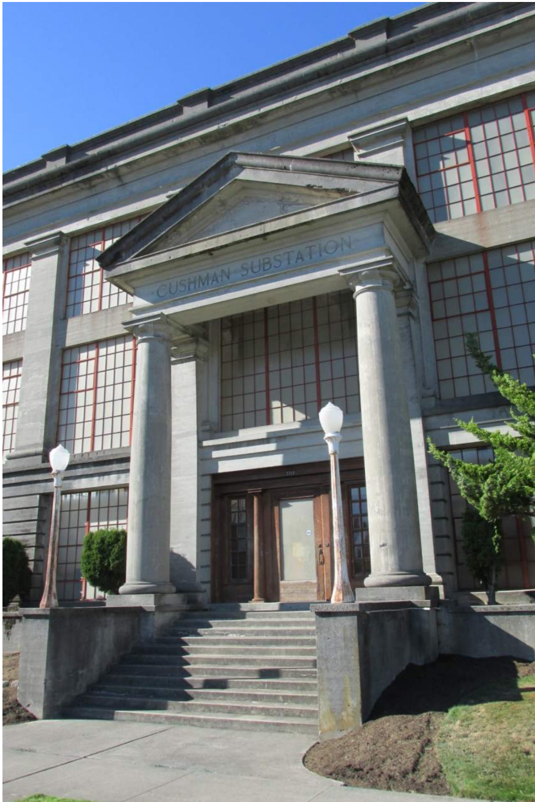
Figure 16 Cushman Substation, main entry onto 19th Street
