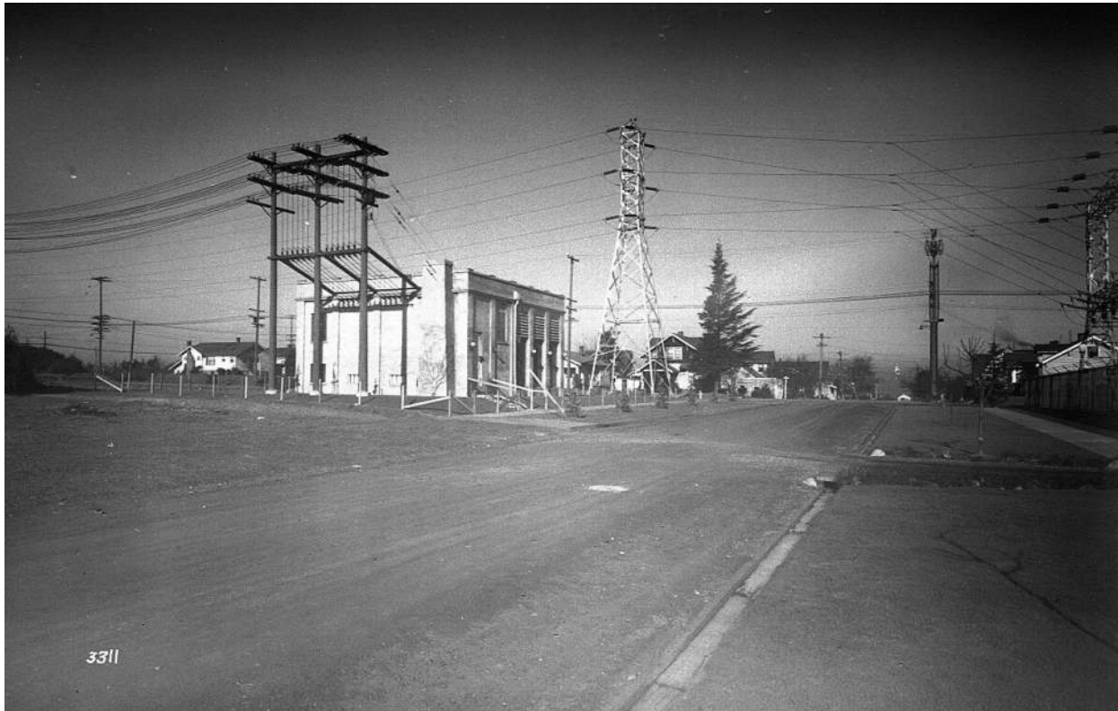
Figure 5. Adams St. Substation, nearly complete, view northwest, 1925. Courtesy of Tacoma Power.
