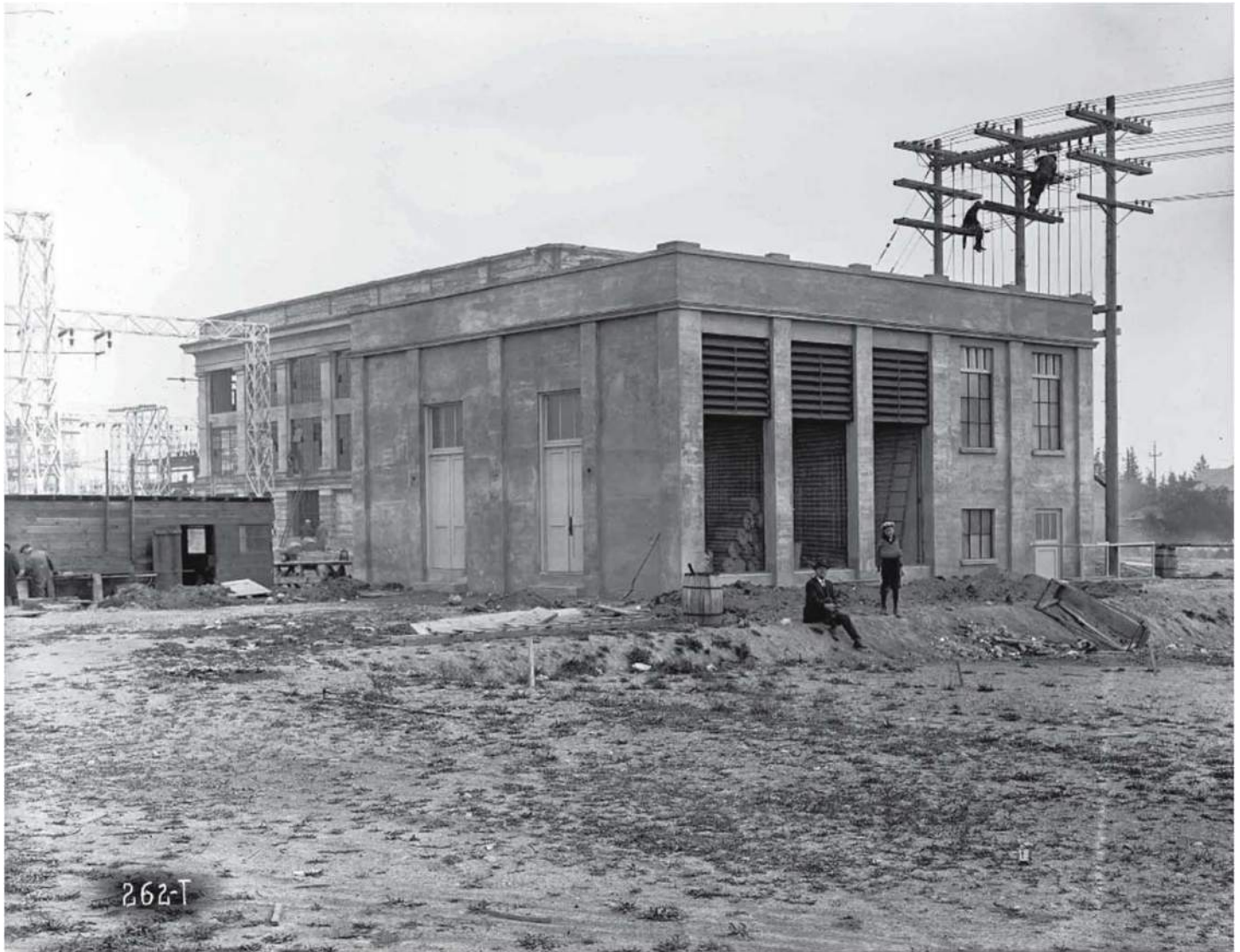
Figure 7 Adams Street Substation; view southeast, October 6, 1925, Image courtesy of Tacoma Power
