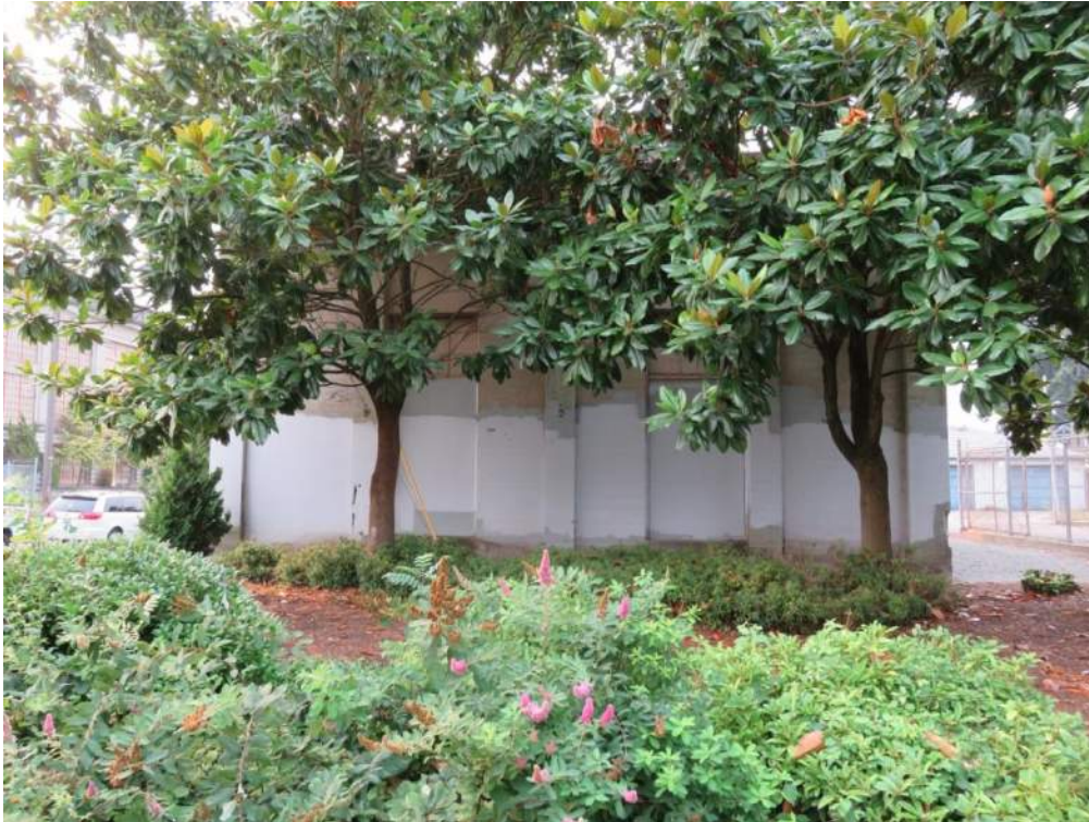
Photo 6 of 13. WA_PierceCounty_AdamsSt.Substation_0006. Adams St. Substation, north elevation, view south.
