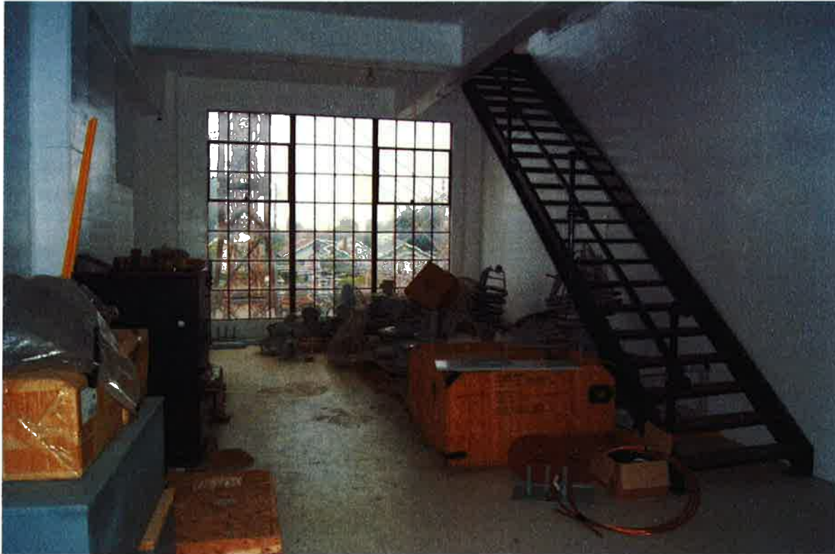
Photo 14 of 17. WA_PierceCounty_CushmanSubstation_0014. Stair from second to third level at Cushman Substation.
