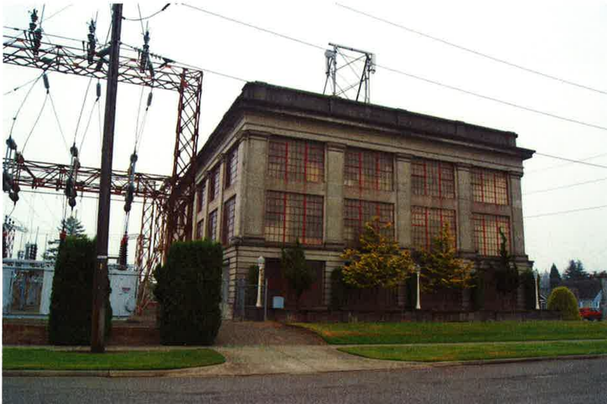
Photo 4 of 17. WA_PierceCounty_CushmanSubstation_0004. Northwest oblique of Cushman Substation, viewing southeast.
