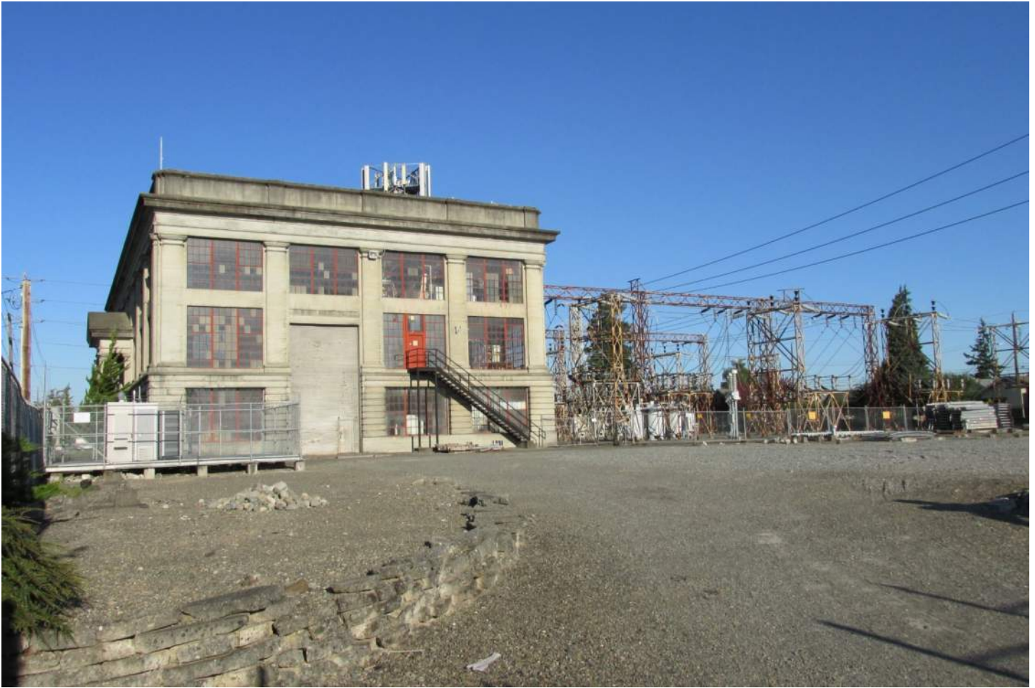
Figure 21 Cushman Substation, view west
