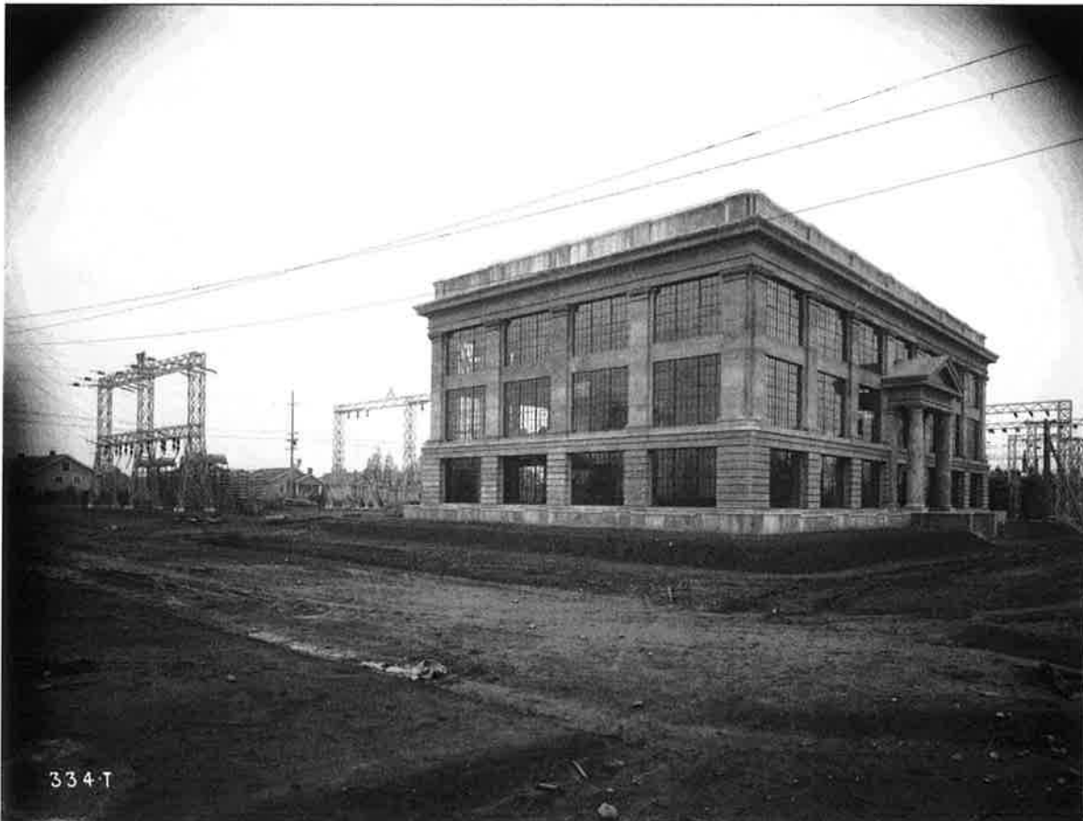
Figure 2. Cushman Substation, 1925, southwest oblique (viewing northeast) with view to switchyard. Image courtesy of Tacoma Power.
