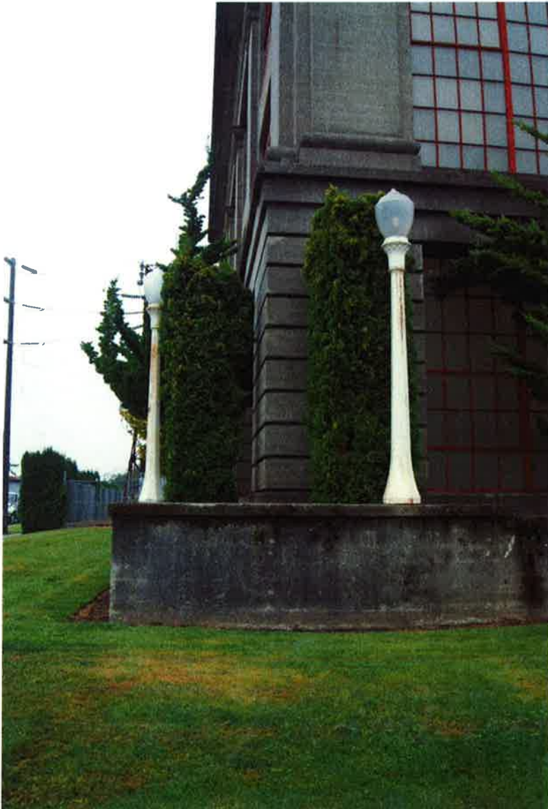
Photo 8 of 17. WA_PierceCounty_CushmanSubstation_0008. Detail of the original cast concrete lamp posts located on the northwest corner of Cushman Substation. The globes are modern plastic.
