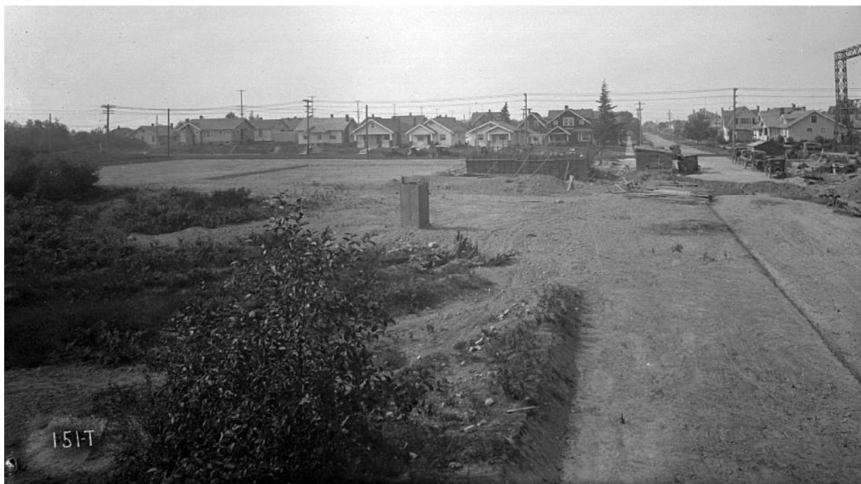
Figure 1. The site of the Adams St. Substation as construction begins, view north, 1925. Courtesy of Tacoma Power.
