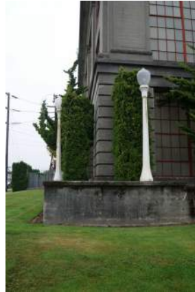
Detail of light poles
